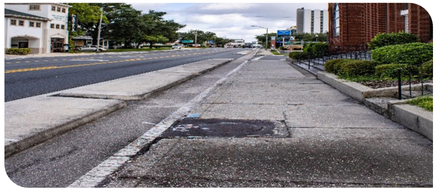
Fig. 5 - Existing drainage structures on SR 37
