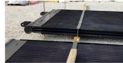
Figure 3: Harps LPECSB & C are staged on 6'x9" cribbing
