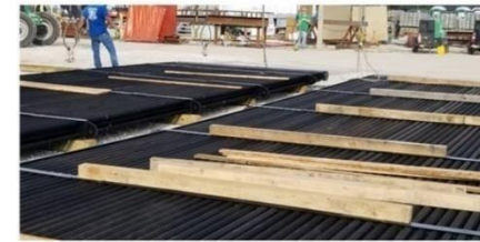
Figure 4: Harps LPECSB & C are staged on 6'x8" cribbing. LPECSA arrived shortly after. LPECSA, B & C will be stacked on top. TEIC intends to stack the harps 5 to 6 high
