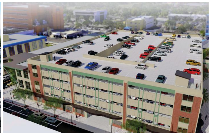
Heritage Parking Garage, lakelandgov.net
