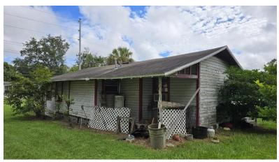
The roofing and roof decking would need to be replaced. The home will not meet any current wind codes because the load paths from the roof rafters to the foundation are not connected. There is no ADA accessibility.
