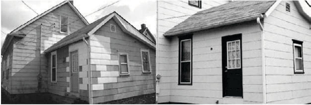
Figure 8.6: Replacement non-asbestos fiber-cement shingles in place, before being painted and after (photo by author).
