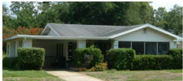
Figure 5.29: Modern Vernacular (Frame and Masonry)
