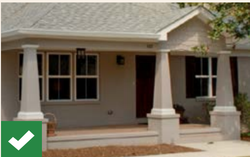
Appropriate Column and Beam Details
