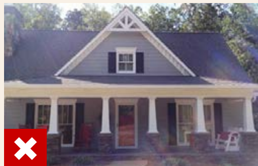
Inappropriate Column Placement: No Window Bay definition
