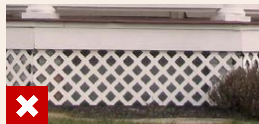
Porch Skirting Without a Frame
