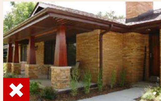
Inappropriate Porch Columns and Beam Details
