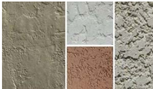
Stucco and Masonry Wall Finishes
