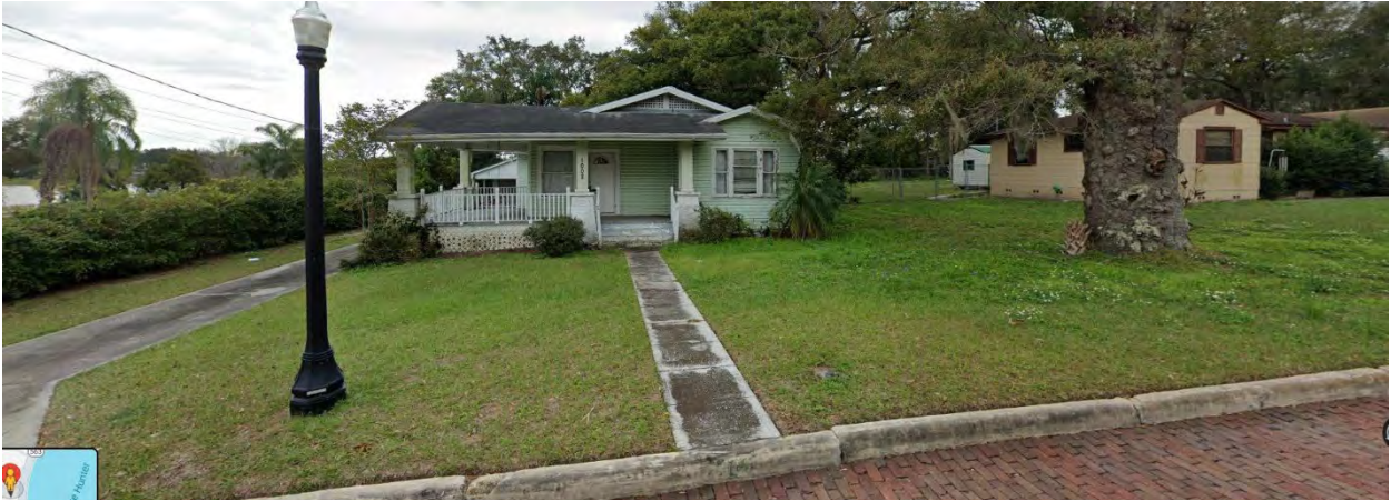
Street view of 1002 Josephine Street
