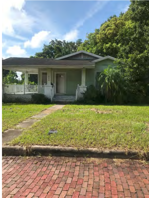
Front view of 1002 Josephine Street
