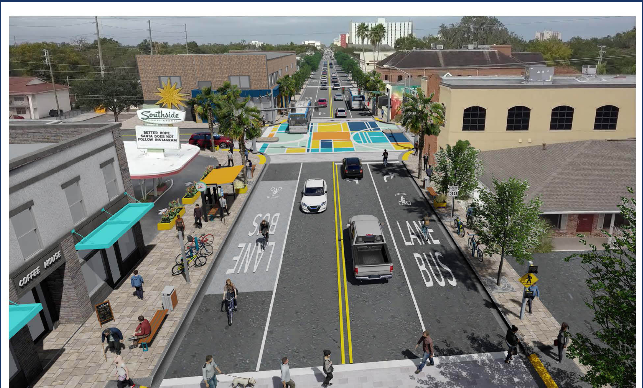
South Florida Avenue & FL Wright Way 4 LANE UNDIVIDED WITH SHARED BUS/BIKE OUTSIDE LANES WITH 6 FT. SIDEWALKS OPTION
