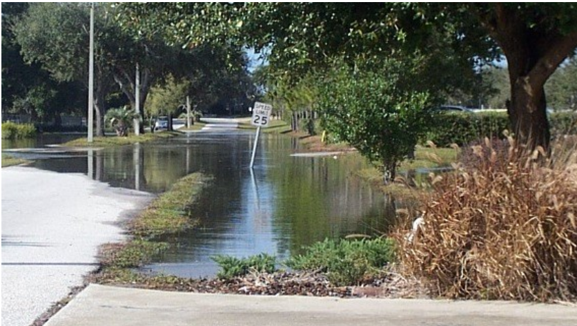
Roadway flooding in North Lakeland
